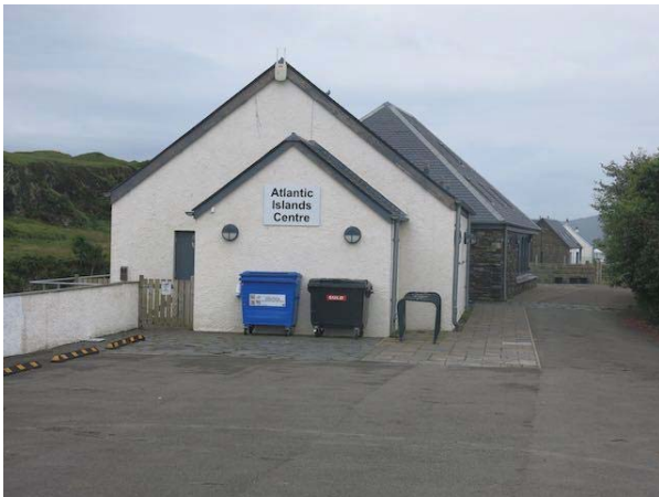
Cullipool's most recent development and a very high profile development within Conservation Area, there is a white wall against white building and stone wall adjoining stone building.
