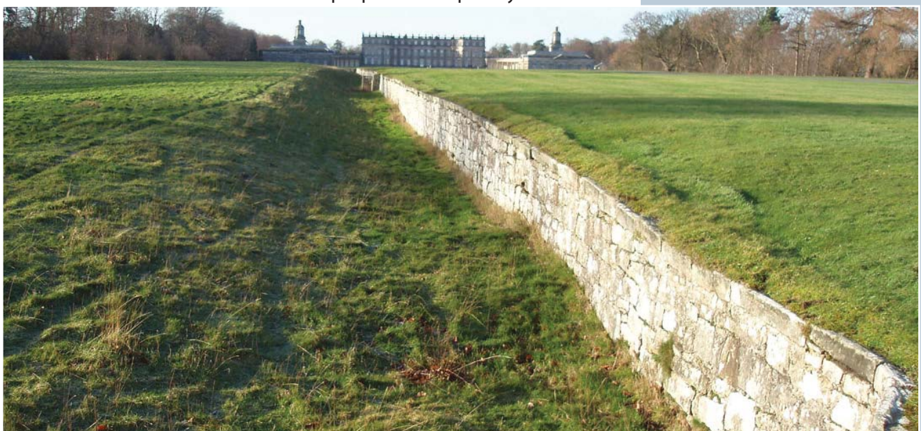
Hopetoun House, West Lothian, viewed from beyond the haha. The sunken wall and ditch allowed unobstructed views from the house, but kept livestock out of the garden.
