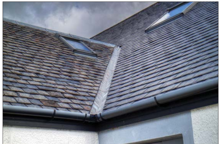
New and reclaimed slates on Community Centre
