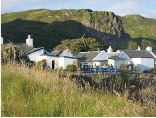
Ellenabeich - South, White rendered shed/store/workshops with black/dark grey roofs. No stone cladding.
