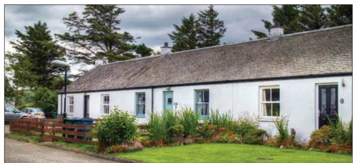
New, inappropriately small, chimneys
