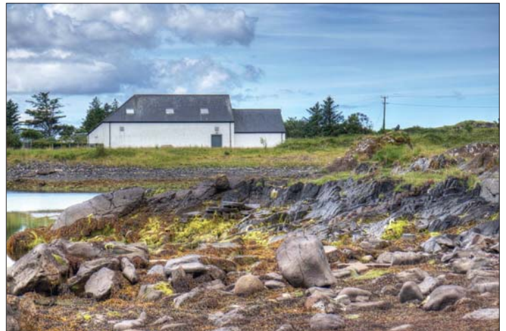
The Community Centre, showing hipped roof
