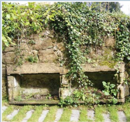
Bee boles (niches for bee hives) set into a boundary wall at Law's Close, High Street, Kirkcaldy, Fife.
