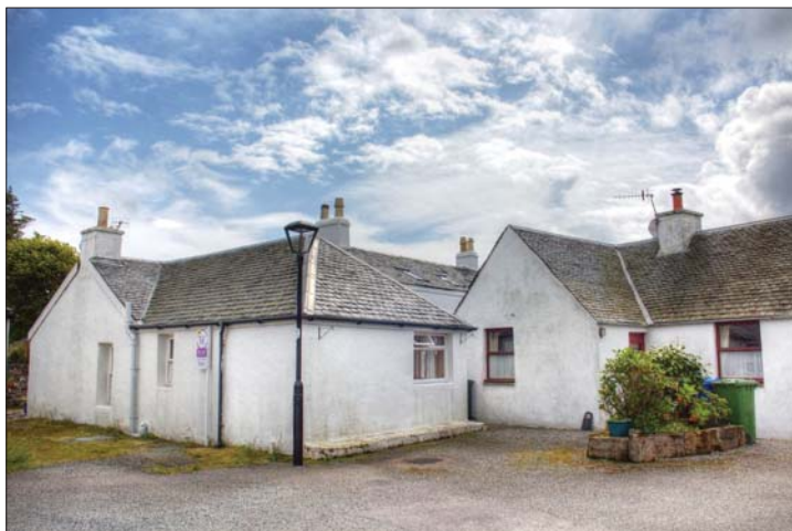
Hipped end of newer extension
