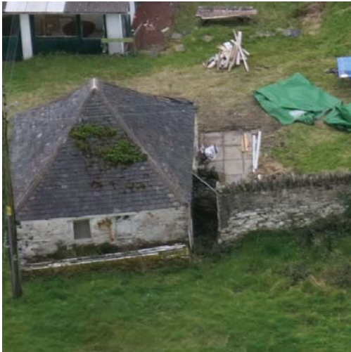
Highland Arts, Ellenabeich - Probably the oldest outbuilding in village, also white rendered/painted. The wall has also been white rendered/painted although weather and time have removed some of this.
